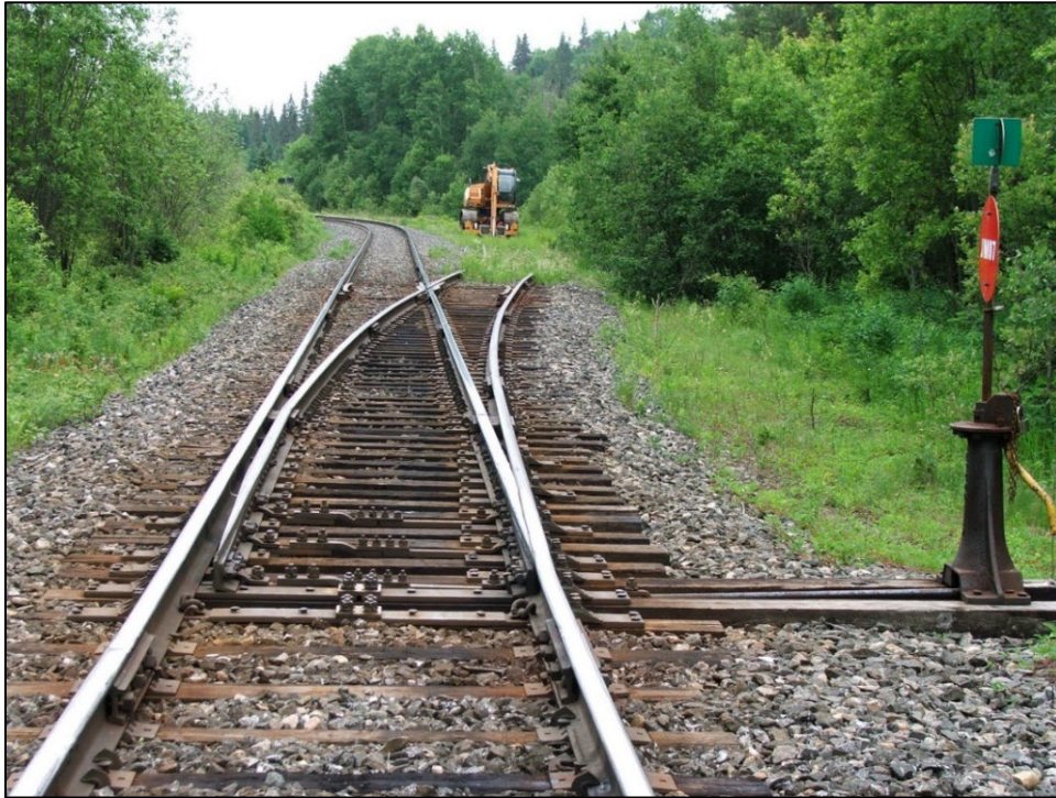
Figure 5. Typical hand-operated switch in an occupancy control system (Source: TSB)
