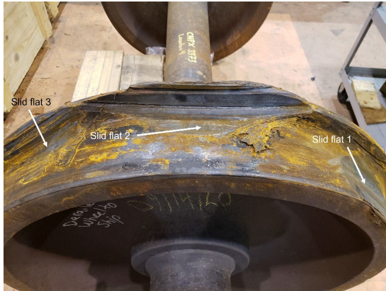
Figure 14. Tread damage on the R4 wheel showing the location of the 3 slid flats (Source: TSB)
