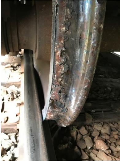
Figure 3. L3 wheel of car CNPX 3373 derailed inside the track gauge of the south rail (Source: Canadian National)
