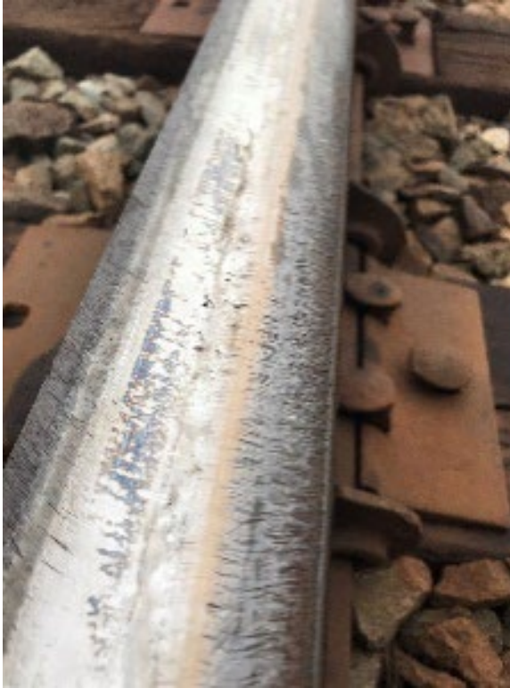
Figure 5. Blueing on the south rail head (Source: Canadian National)
