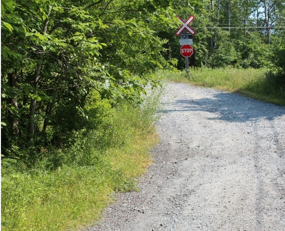
Figure 4. Southward approach to crossing (Source: TSB)
