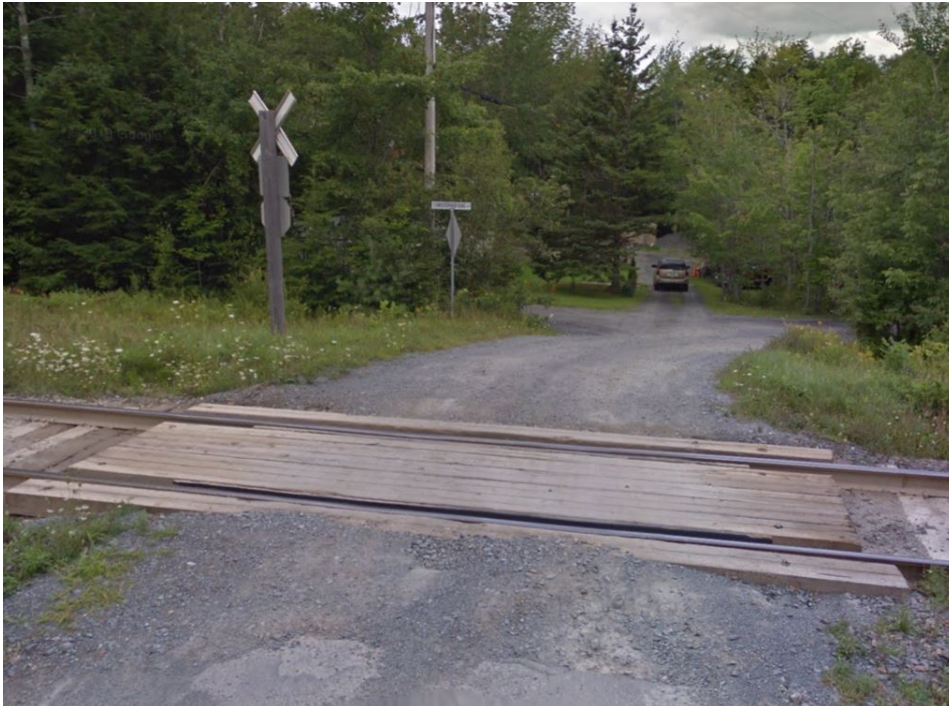
Figure 3. Crossing surface looking north (Source: Google Maps Street View)
