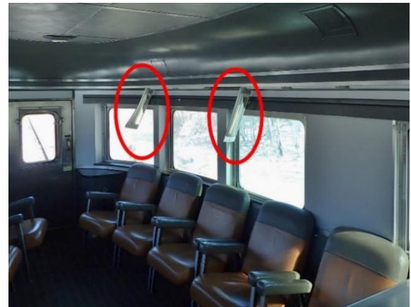
Figure 8. Partially dislodged ceiling panels on VIA 8711 (Source: TSB)
