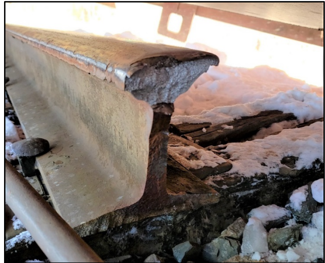
Figure 3. Broken, partly worn rail at Mile 103.73 (Source: TSB)
