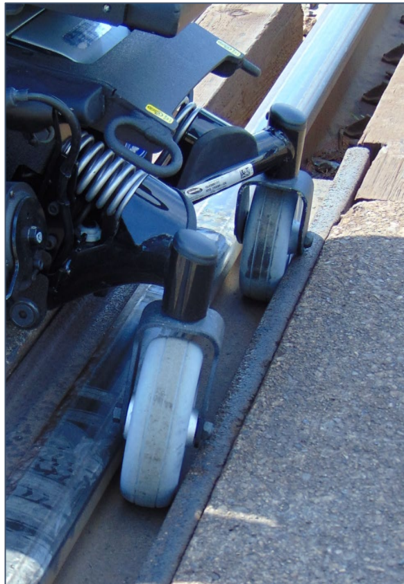
Figure 6. Rear caster wheels of exemplar wheelchair lodged in the flangeway gap at the occurrence crossing (Source: Royal Canadian Mounted Police)
