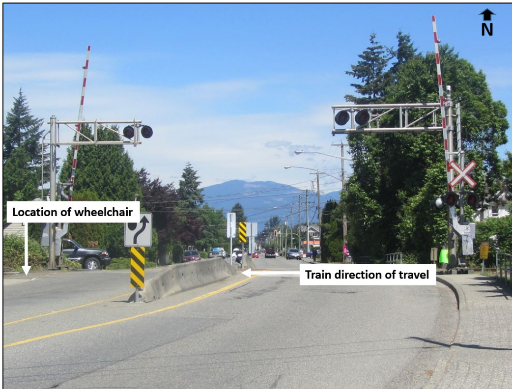
Figure 5. Street view of Broadway Street public crossing, looking north (Source: TSB)
