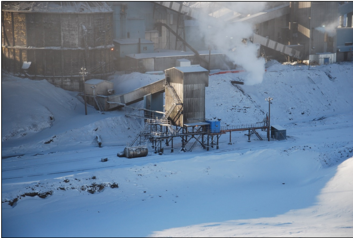
Figure 2. Coal loading facility at the Luscar Mine (Source: TSB)
