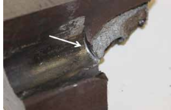
Photo 5. Deformation from joint bar contact at the fillet under the head on the field side of rail piece No. 1 (arrow)
