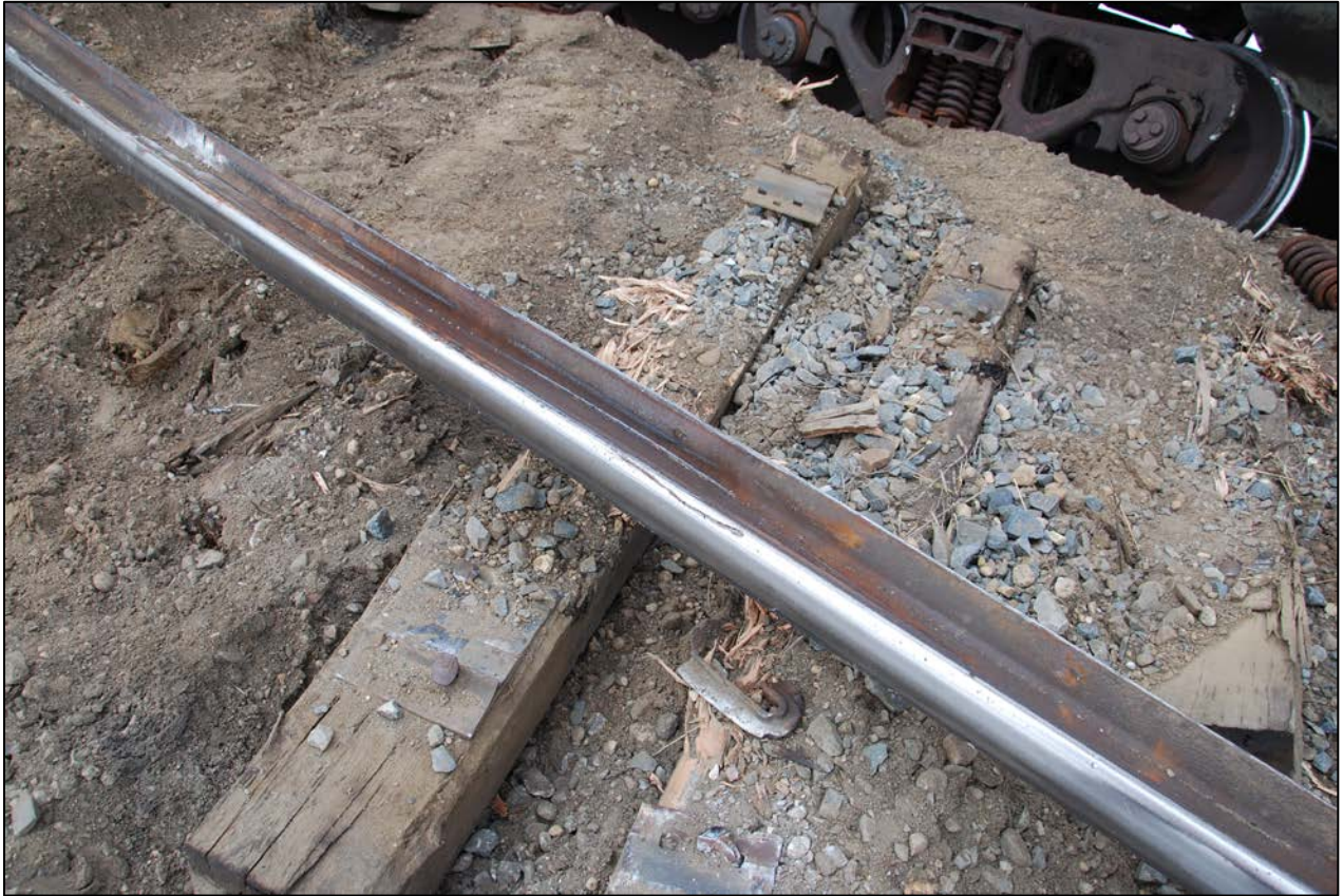
Photo 5. Subgrade and ballast conditions near the POD
