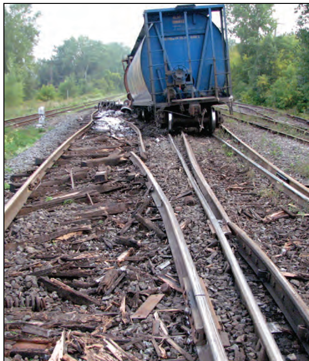
Photo 1. Damage to tracks and turnouts
