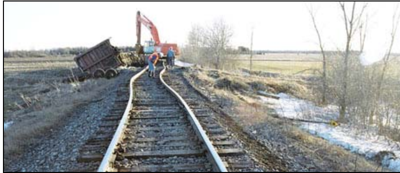
Photo 1. Southward view showing the track buckle and derailment
