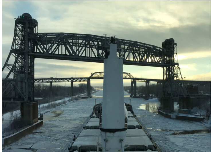
Figure 3. Seaway bridges 7A and 7B with spans lifted, downbound view. The Honoré-Mercier Bridge is visible in the background. (Source: third party, with permission)
