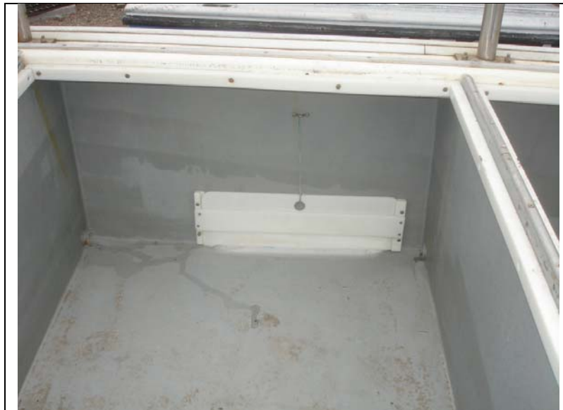
Photo 6. Slider style freeing port viewed from inside vessel
