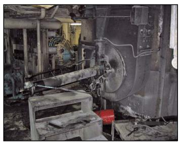
Photo 7. External damage to starboard auxiliary boiler
