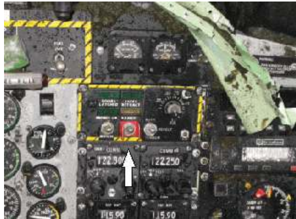
Figure 2 - System indicating lights and door armed switch (indicated by white arrow) in the On position
