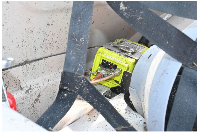
Figure 5. The occurrence aircraft's ARTEX ELT 1000 installation, looking aft at the right side of the baggage compartment, behind the right seat (Source: TSB)
