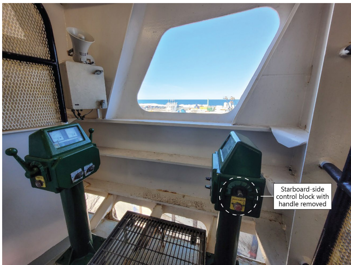
Figure 5. View of the starboard-side control station showing control blocks for the port-side equipment (left) and starboard-side equipment (right) (Source: TSB)
