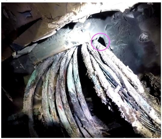
Figure 19. Unsealed deck penetration (circled) (Source: TSB)
