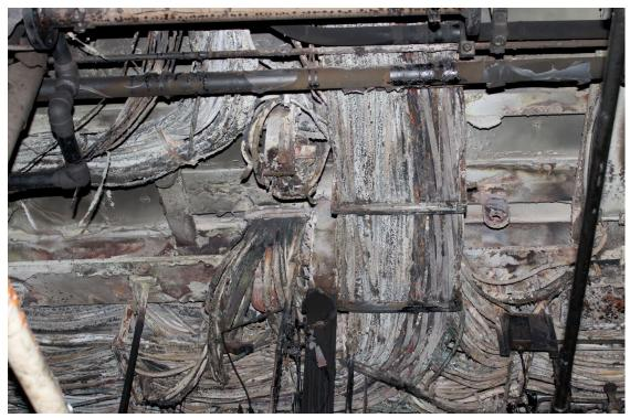
Figure 10. Burned electrical cables running along the underside of the 24-foot flat (Source: TSB)
