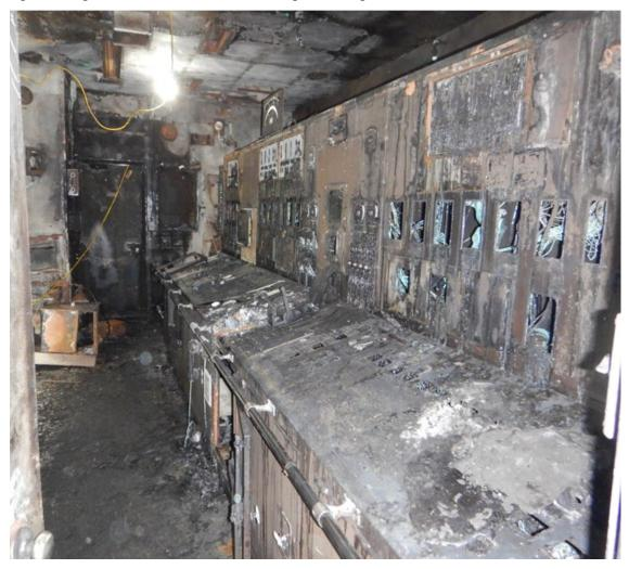
Figure 11. Engine control room consoles, showing fire damage (Source: TSB)
