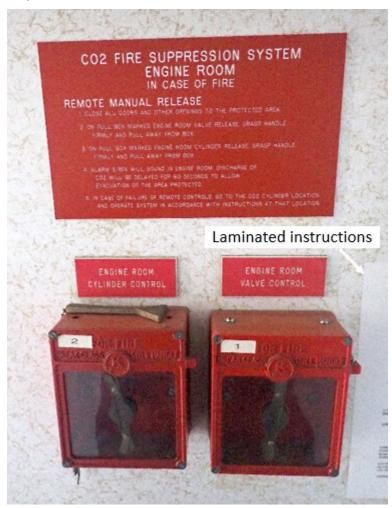
Figure 13. Tecumseh's  $CO_2$  remote release station on deck C (Source: TSB)
