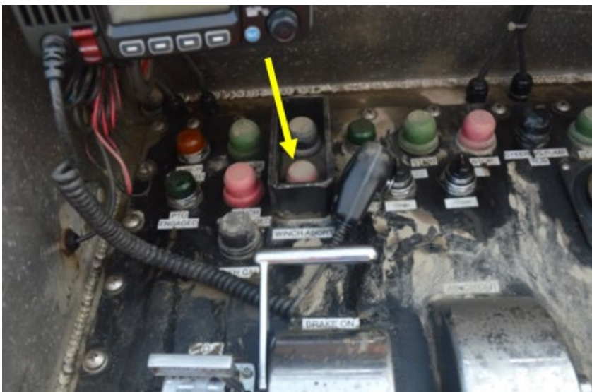
Figure 9. Abort mechanism at the conning station on the upper aft deck, with the abort button indicated by a yellow arrow (Source: TSB)
