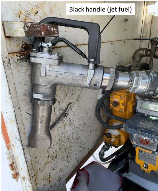
Figure 5. Spout for jet fuel, identified by black handle (Source: North Star Air Ltd., with TSB annotations)
